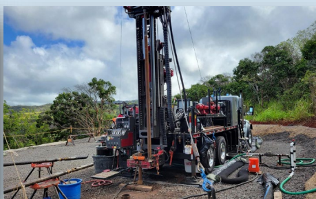
Drilling additional groundwater monitoring wells to increase visibility
