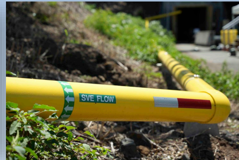
Soil vapor extraction pilot study to evaluate remediation technology
